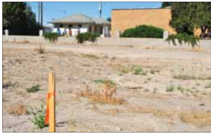
Wood stakes marked with orange caution tape indicate the footprint of the library expansion would be located to the east of the current Homedale Public Library.
